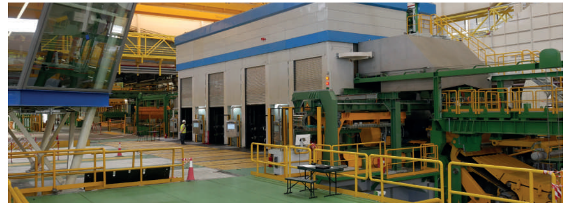
Four-stand Tandem hot finishing mill - Aluminium segment
