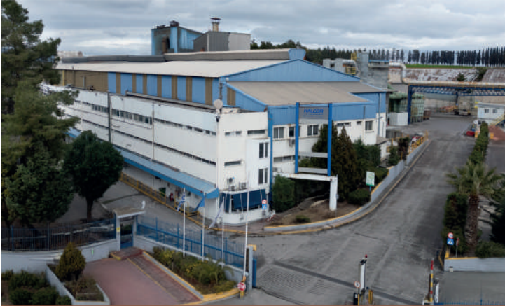
Foundry | Oinofyta, Greece
