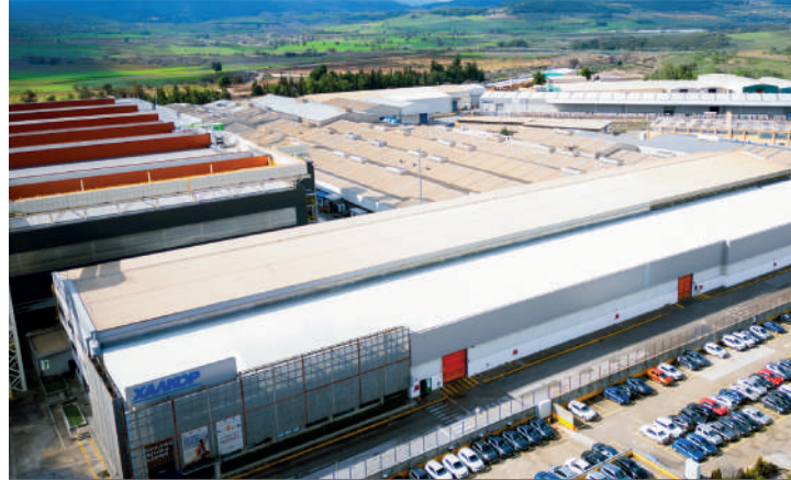
Copper Tubes | Oinofyta, Greece
