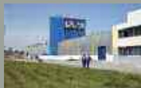
Hellenic Cables Livadia, Greece
